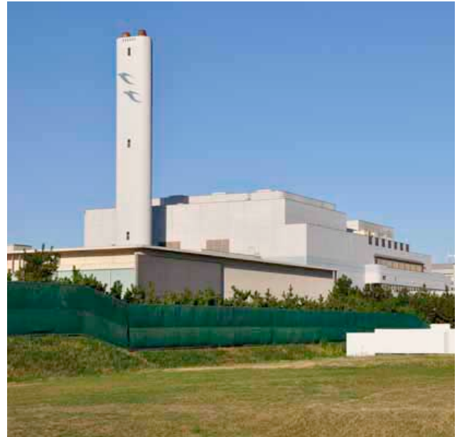
Waste Incinerator in Japan (Photo by Gerald)
